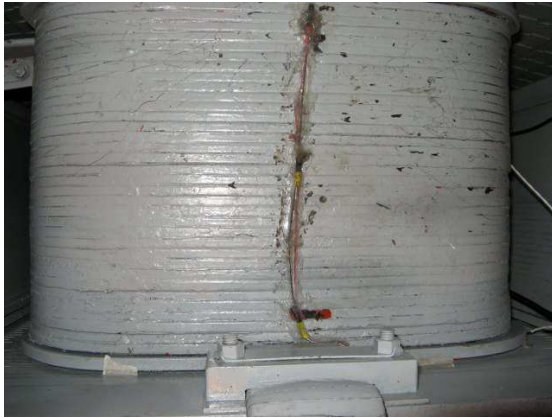
Fig. 9. Temperature sensors glued to rotor pole winding in HPP Dubrovnik. All sensors are mutually connected in parallel and end up with one transmitter/receiver.
