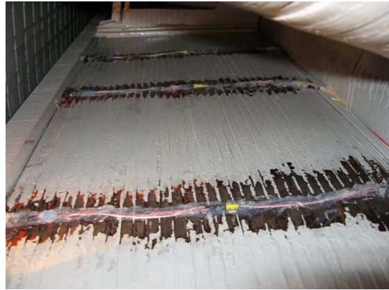
Fig. 9. Temperature sensors glued to rotor pole winding in HPP Dubrovnik. All sensors are mutually connected in parallel and end up with one transmitter/receiver.
